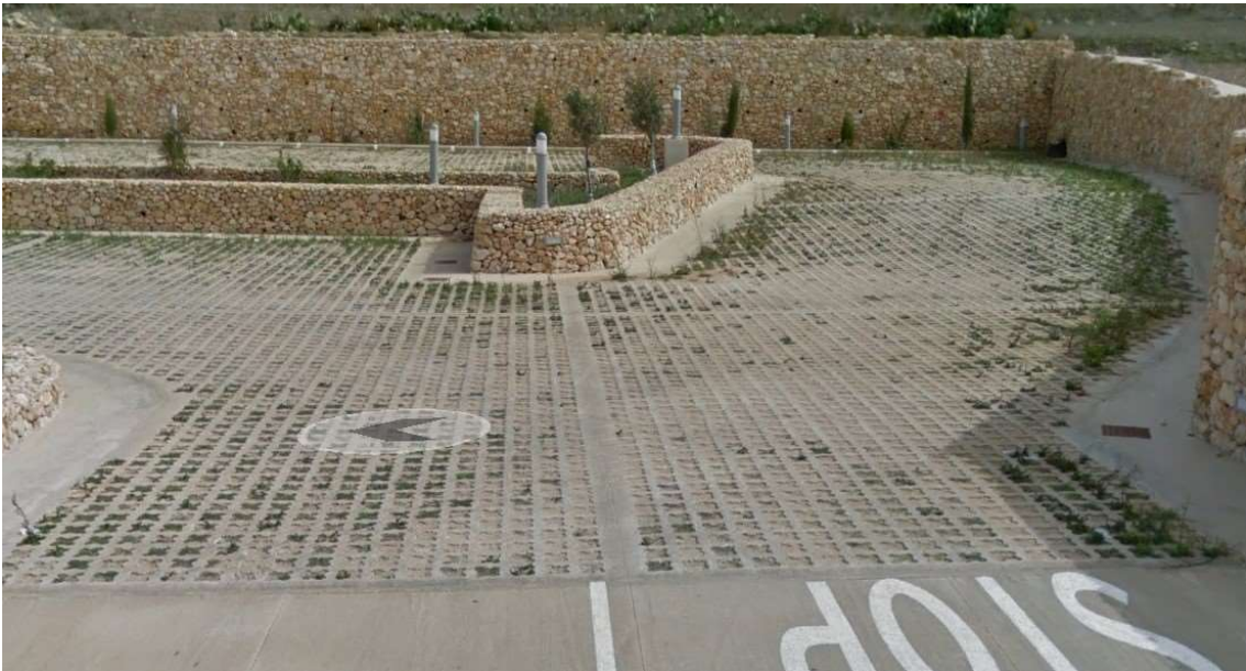
Figure 80: Permeable pavement at Għarb, Gozo
