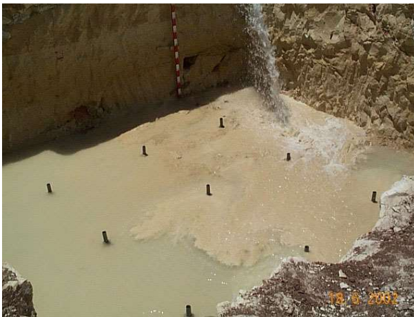
Figure 61: Borehole wells at MDH soakaway under test
