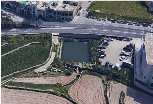
Figure 19: Soakaway at Żebbuġ
