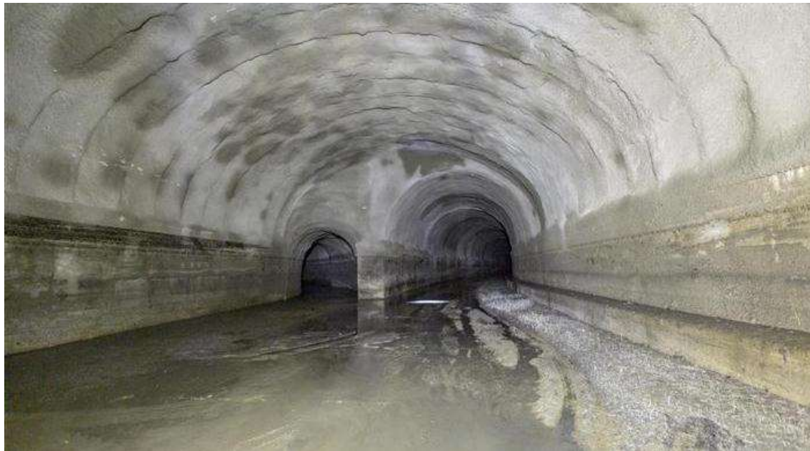
Figure 31: NFRP internal view of a tunnel confluence
