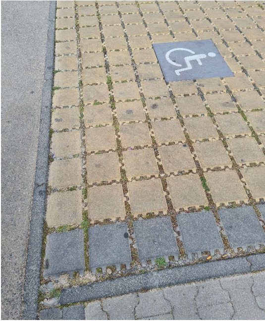
Figure 78: Permeable pavement at Mosta
